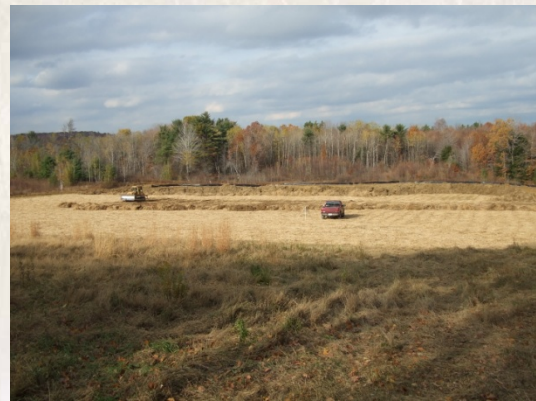
Wetland under construction
