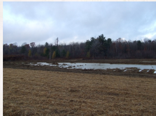
Completed wetland basin prior to seeding
